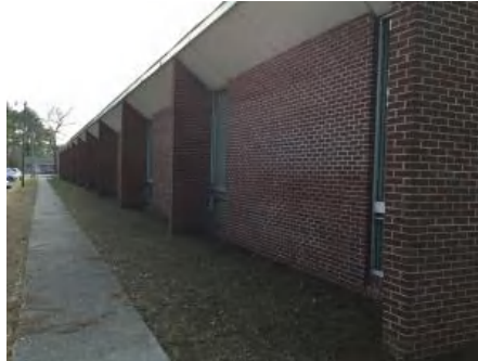
2). West Elevation - Feb 16, 2017
