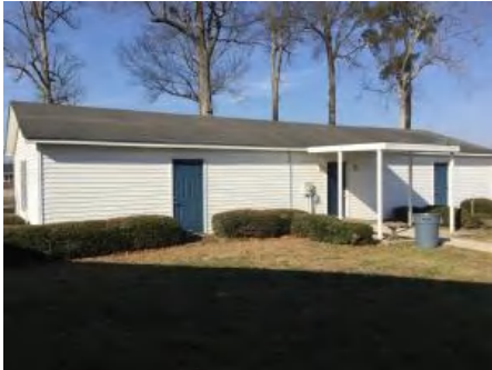
1). East Elevation - Feb 13, 2017
