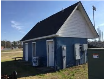
4). East Elevation - Feb 16, 2017
