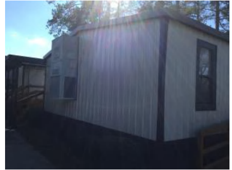
3). West Elevation - Feb 10, 2017
