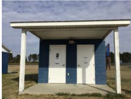
2). North Elevation - Feb 22, 2017
