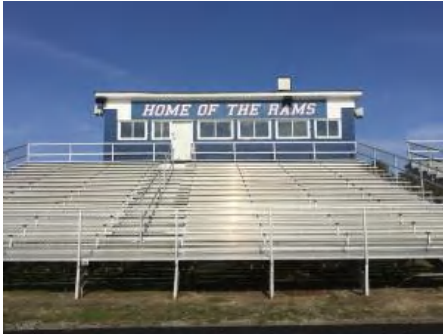
1). South Elevation - Feb 16, 2017
