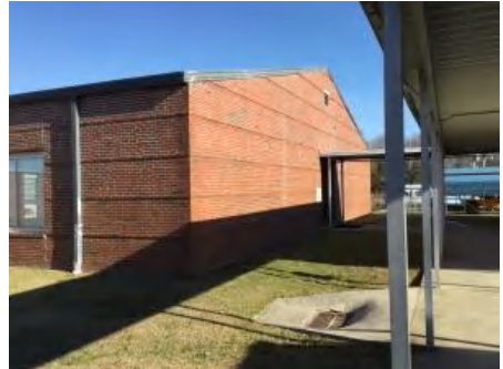
3). Southeast Elevation - Feb 13, 2017
