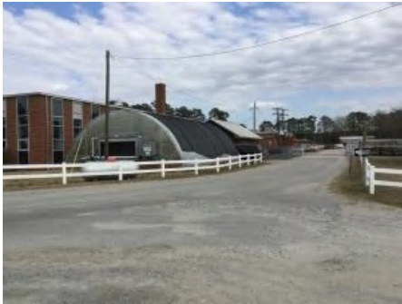
4). East Elevation - Feb 16, 2017
