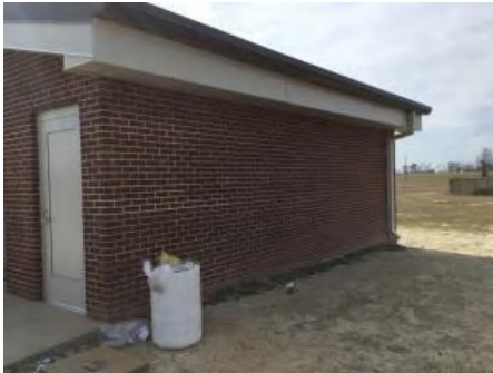
4). North Elevation - Feb 22, 2017
