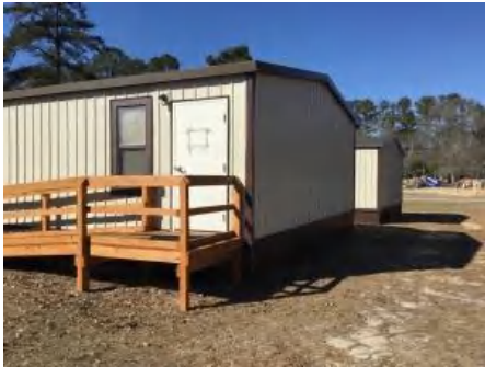
4). East Elevation - Feb 10, 2017
