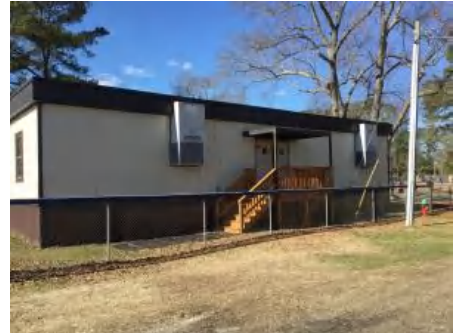
3). East Elevation - Feb 13, 2017
