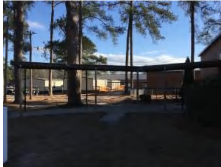
2). North Elevation - Feb 13, 2017
