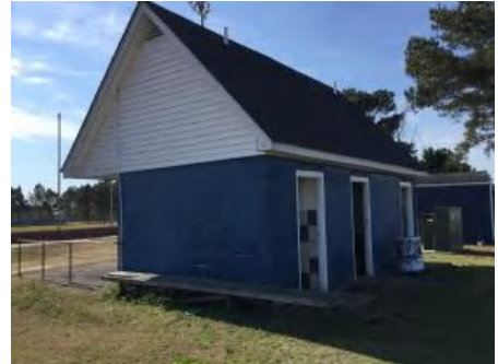
3). North Elevation - Feb 16, 2017
