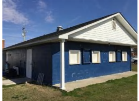
3). West Elevation - Feb 16, 2017
