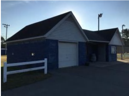
1). North Elevation - Feb 17, 2017
