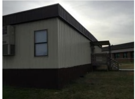
3). West Elevation - Feb 22, 2017
