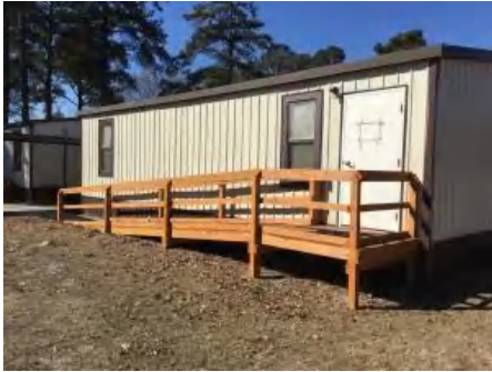
1). North Elevation - Feb 01, 2017
