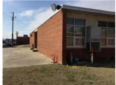
3). South Elevation - Feb 16, 2017
