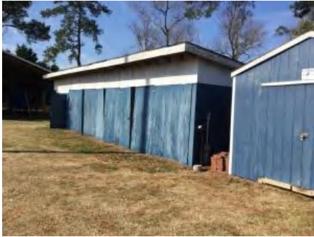
1). East Elevation - Feb 23, 2017
