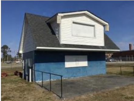
1). South Elevation - Feb 16, 2017
