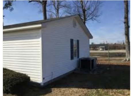
3). North Elevation - Feb 13, 2017
