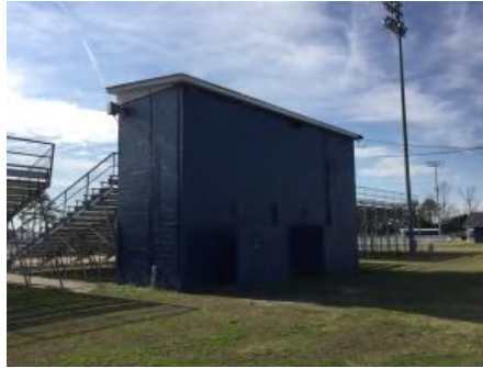
2). Northwest Elevation - Feb 16, 2017
