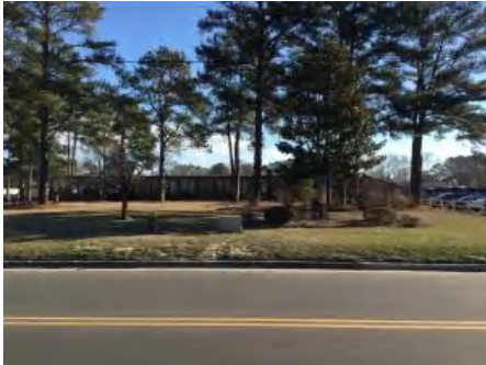
1). West Elevation - Feb 13, 2017
