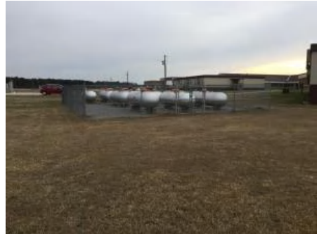
3). East Elevation - Feb 22, 2017
