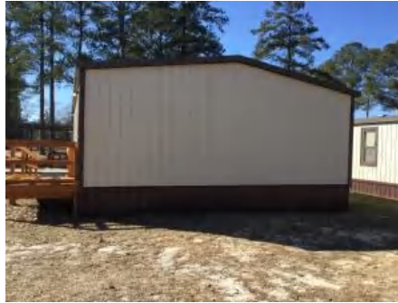
2). West Elevation - Feb 01, 2017
