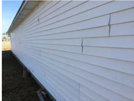
2). West Elevation - Feb 23, 2017
