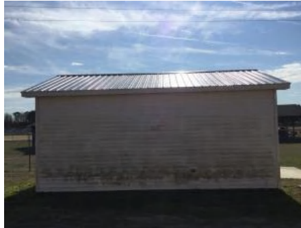
2). North Elevation - Feb 23, 2017
