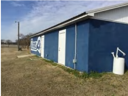
1). South Elevation - Feb 22, 2017
