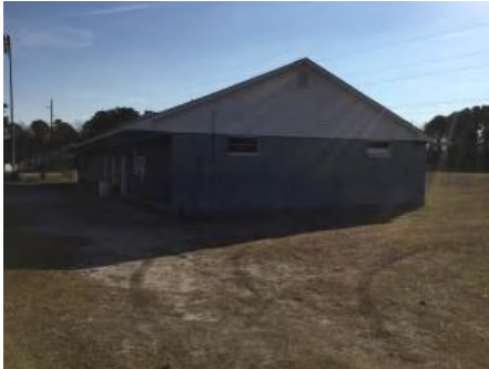
1). North Elevation - Feb 13, 2017
