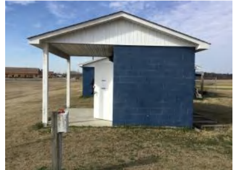
3). East Elevation - Feb 22, 2017
