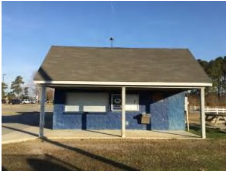
4). South Elevation - Feb 17, 2017
