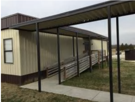
1). East Elevation - Feb 22, 2017
