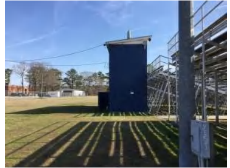
3). East Elevation - Feb 16, 2017
