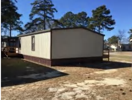
4). Southwest Elevation - Feb 01, 2017
