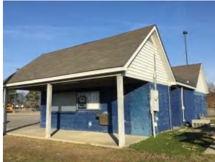
2). West Elevation - Feb 17, 2017
