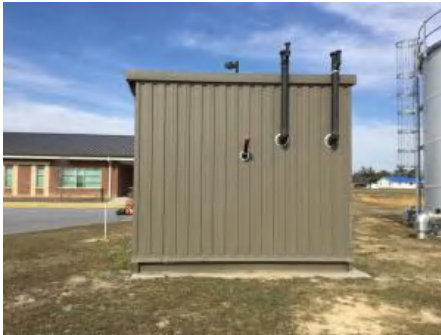
4). South Elevation - Feb 21, 2017
