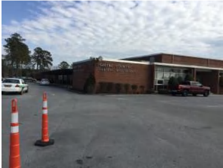
1). North Elevation - Feb 16, 2017
