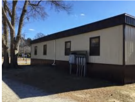
2). North Elevation - Feb 13, 2017
