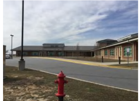
3). Southwest Elevation - Feb 21, 2017
