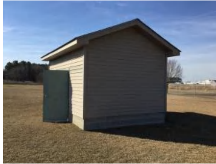
2). East Elevation - Feb 23, 2017
