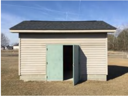
1). North Elevation - Feb 23, 2017
