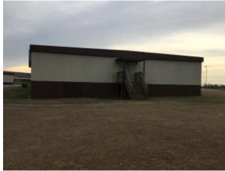
2). West Elevation - Feb 22, 2017
