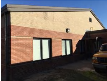
1). South Elevation - Feb 22, 2017
