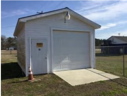
1). West Elevation - Feb 23, 2017
