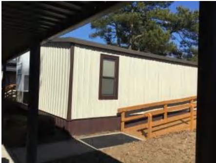
4). East Elevation - Feb 01, 2017
