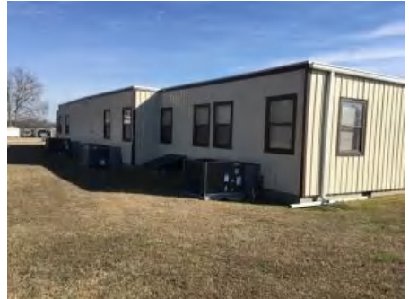
3). North Elevation - Feb 15, 2017
