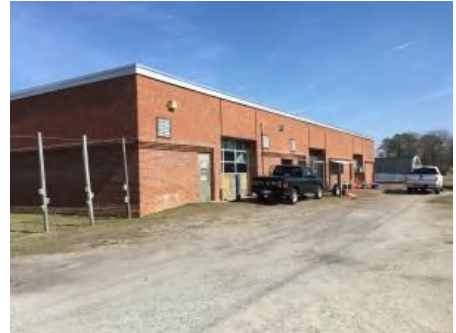
3). West Elevation - Feb 13, 2017
