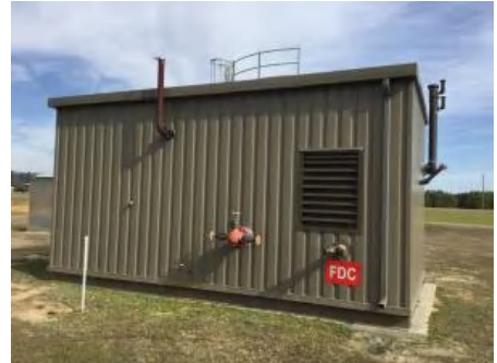
3). West Elevation - Feb 21, 2017
