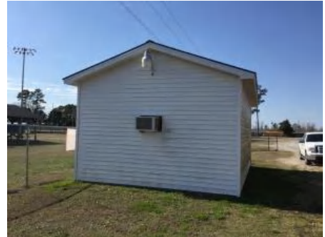
3). East Elevation - Feb 23, 2017
