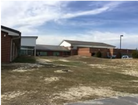
4). Northwest Elevation - Feb 21, 2017
