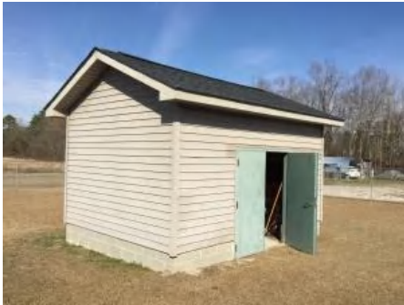
4). West Elevation - Feb 23, 2017
