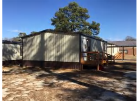
3). East Elevation - Feb 10, 2017
