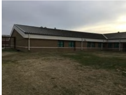
2). West Elevatrion - Feb 22, 2017
