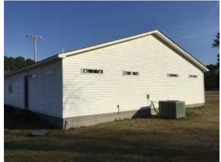
3). North Elevation - Feb 23, 2017
