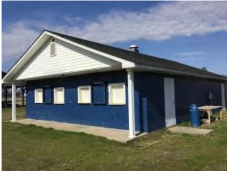
1). East Elevation - Feb 23, 2017
