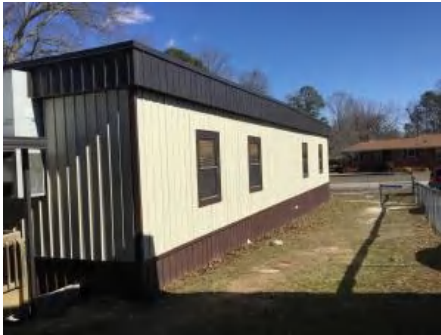
4). South Elevation - Feb 13, 2017
