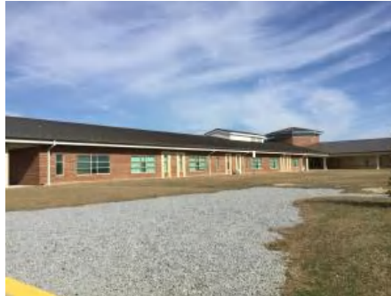
2). Southeast Elevation - Feb 21, 2017
