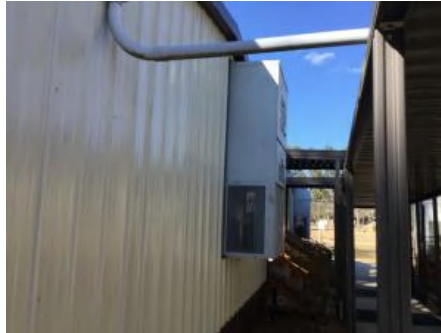
2). West Elevation - Feb 10, 2017
