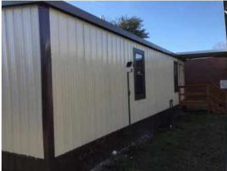
1). Northwest Elevation - Feb 13, 2017
