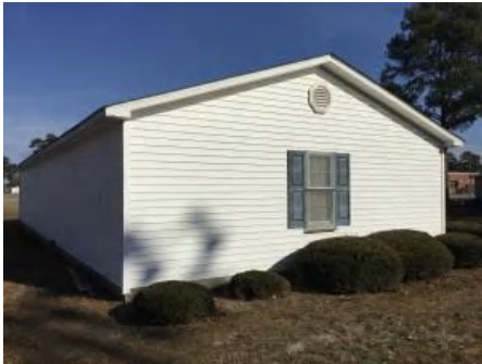
4). Southwest Elevation - Feb 13, 2017
