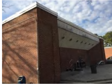
2). East Elevation - Feb 16, 2017
