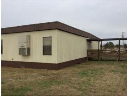
1). East Elevation - Feb 22, 2017
