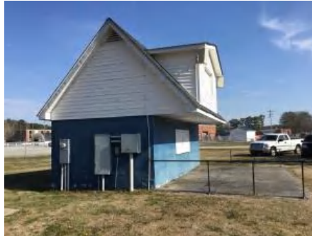
2). West Elevation - Feb 16, 2017
