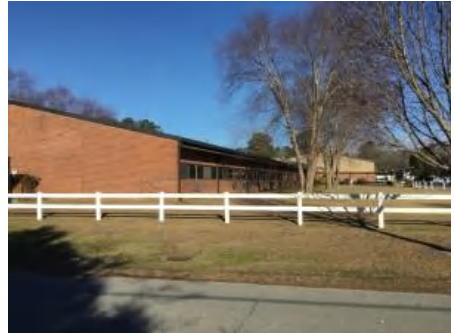
3). East Elevation - Feb 13, 2017
