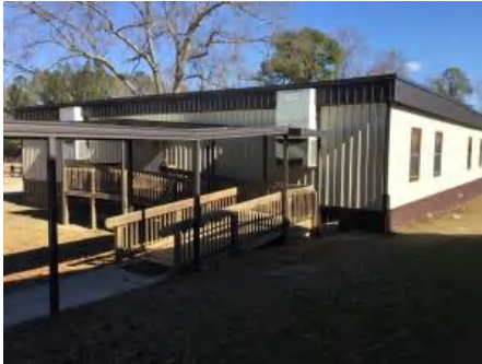
1). West Elevation - Feb 13, 2017
