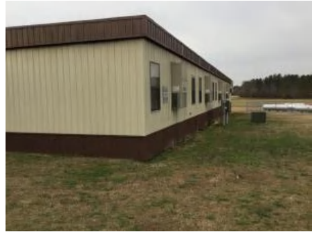
3). North Elevation - Feb 22, 2017
