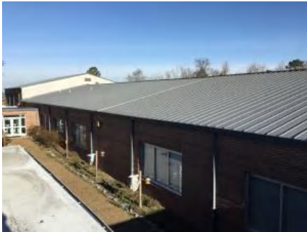
4). Northwest Elevation - Feb 13, 2017
