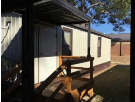
1). North Elevation - Feb 10, 2017
