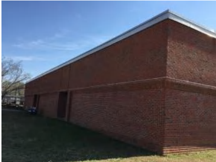
1). North Elevation - Feb 13, 2017
