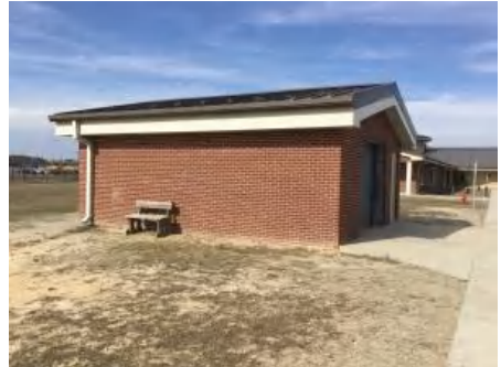
3). South Elevation - Feb 22, 2017
