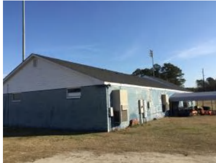
2). East Elevation - Feb 13, 2017
