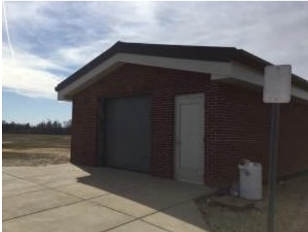
1). East Elevation - Feb 22, 2017
