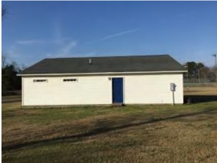
1). East Elevation - Feb 13, 2017
