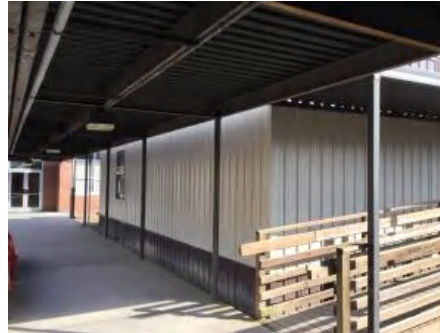
2). West Elevation - Feb 17, 2017
