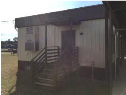
4). East Elevation - Feb 17, 2017
