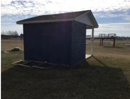
4). South Elevation - Feb 22, 2017
