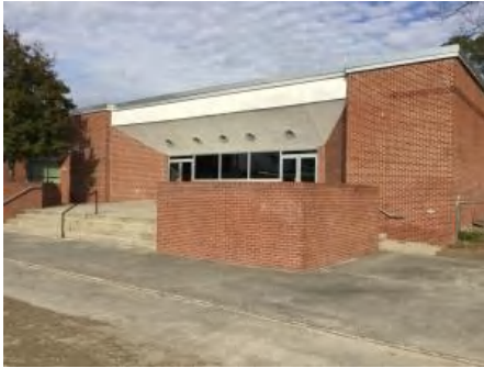
1). West Elevation - Feb 16, 2017
