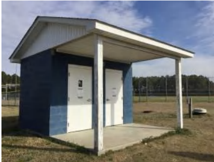
1). Northwest Elevation - Feb 22, 2017
