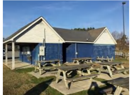
3). East Elevation - Feb 17, 2017
