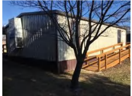
3). Southwest Elevation - Feb 13, 2017
