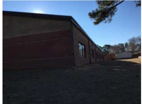
3). West Elevation - Feb 22, 2017
