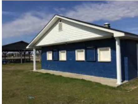
2). North Elevation - Feb 16, 2017
