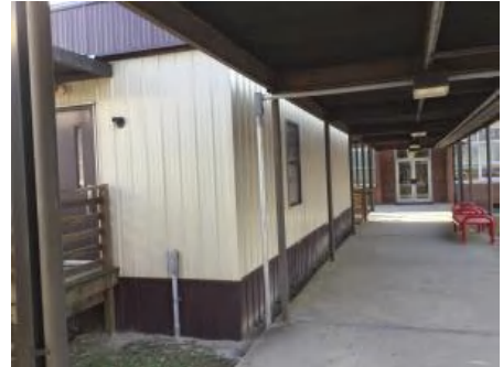
3). North Elevation - Feb 17, 2017
