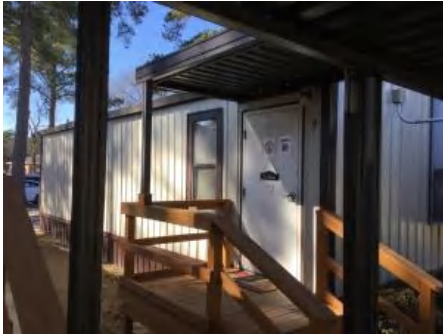
1). North Elevation - Feb 10, 2017
