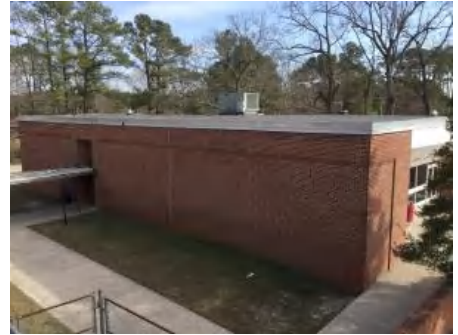
3). North Elevation - Feb 16, 2017
