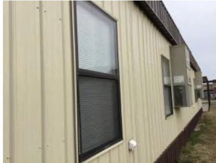
2). South Elevation - Feb 22, 2017
