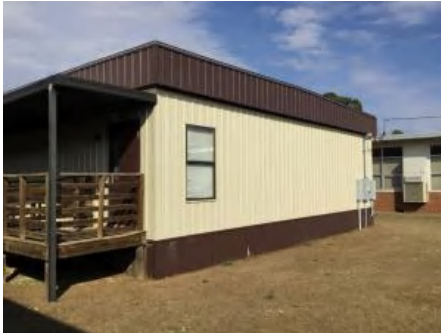
1). South Elevation - Feb 17, 2017
