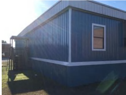
2). Northwest Elevation - Feb 13, 2017
