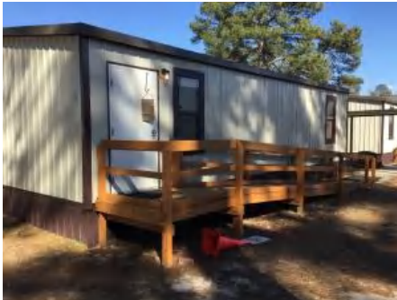
4). North Elevation - Feb 10, 2017
