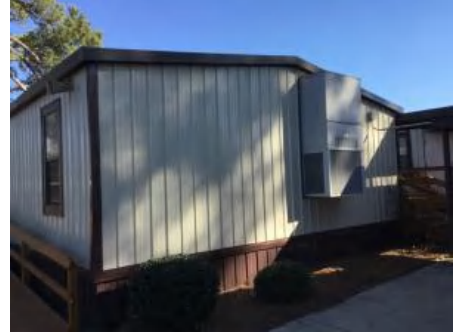
3). East Elevation - Feb 10, 2017
