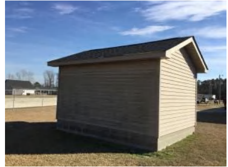
3). South Elevation - Feb 23, 2017
