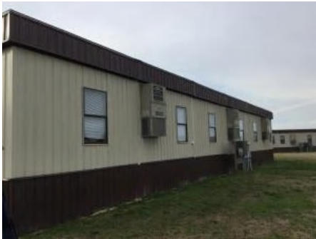
4). North Elevation - Feb 22, 2017
