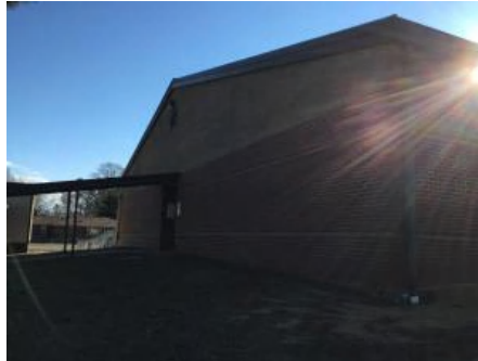
2). North Elevation - Feb 22, 2017
