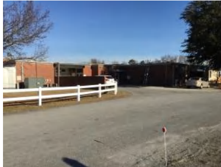
2). East Elevation - Feb 13, 2017
