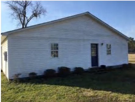
4). West Elevation - Feb 13, 2017
