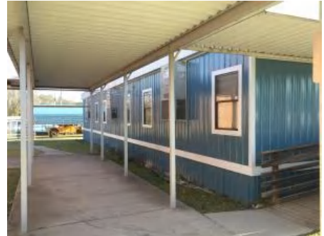
3). Southeast Elevation - Feb 13, 2017
