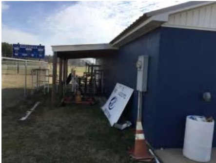
4). North Elevation - Feb 22, 2017
