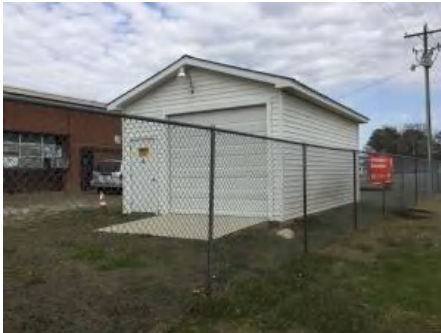
4). South Elevation - Feb 23, 2017
