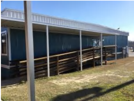
4). Southwest Elevation - Feb 13, 2017
