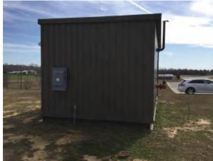
2). North Elevation - Feb 21, 2017
