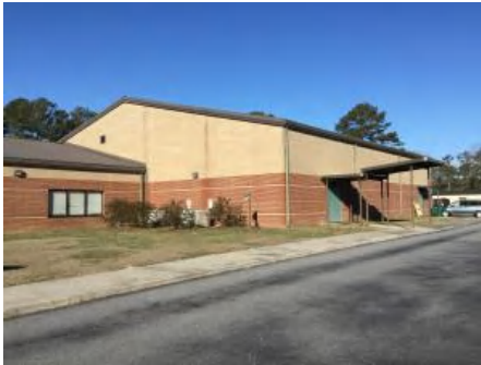
4). East Elevation - Feb 13, 2017
