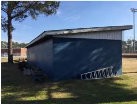
4). North Elevation - Feb 16, 2017
