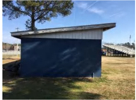
3). West Elevation - Feb 16, 2017
