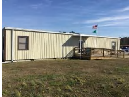
2). West Elevation - Feb 15, 2017
