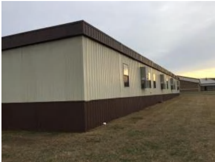
4). South Elevation - Feb 22, 2017
