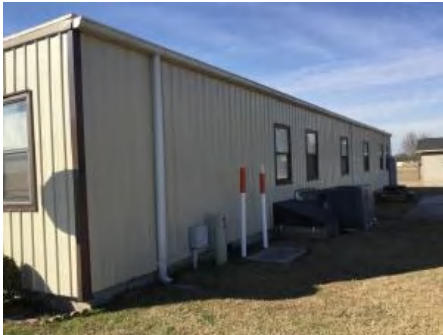
4). East Elevation - Feb 15, 2017
