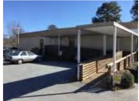
3). North Elevation - Jan 31, 2017
