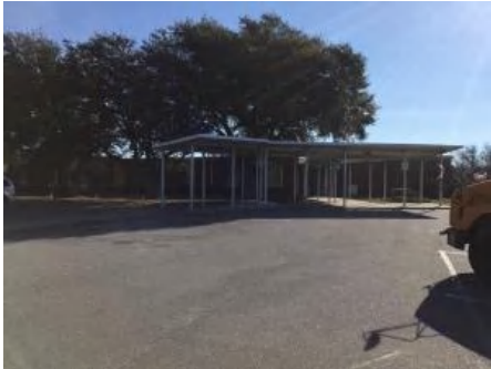
1). West Elevation - Feb 13, 2017
