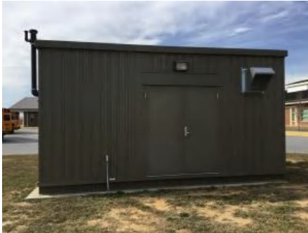
1). East Elevation - Feb 21, 2017
