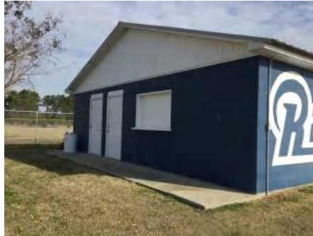
2). East Elevation - Feb 22, 2017
