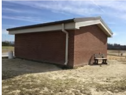
2). West Elevation - Feb 22, 2017
