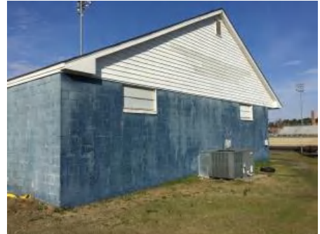
3). West Elevation - Feb 13, 2017
