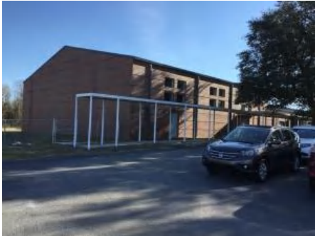
1). Northwest Elevation - Feb 13, 2017
