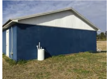
3). West Elevation - Feb 22, 2017
