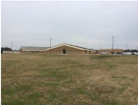
4). North Elevation - Feb 22, 2017
