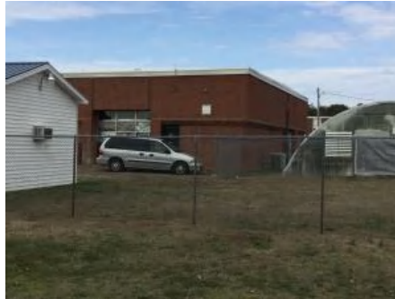
2). East Elevation - Feb 13, 2017
